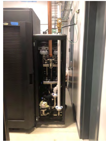
Figure 3.23. Server Room Chiller installation.
