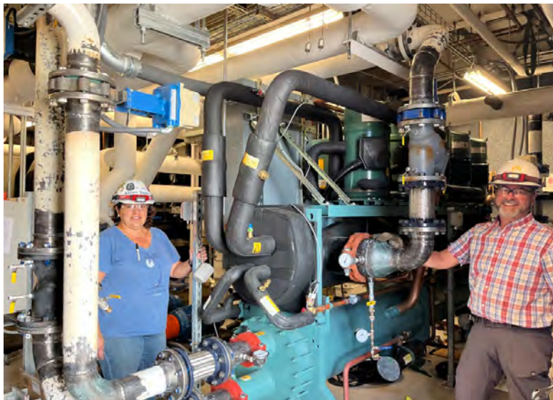
Figure 3.18. Replacement Chiller #1 ready for commissioning.
