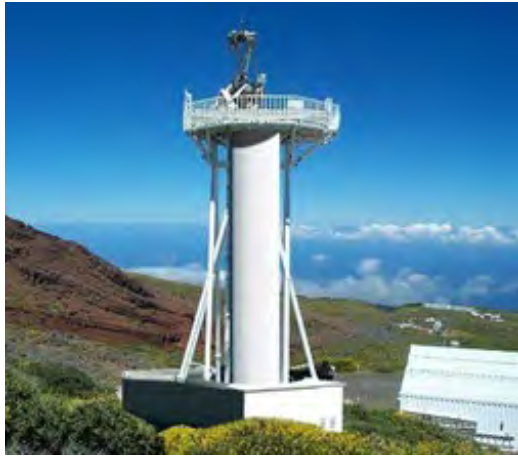
Figure 4-11. A potential concept of an ngGONG site with the telescopes in a fully retractable dome (shown open here), a structural element containing the transfer optics, and the base building.
