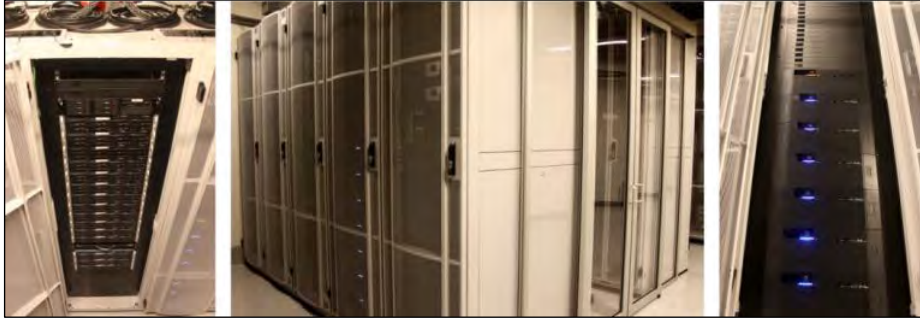
Figure 6-8. Photos of the NISP Data Center in Boulder showing the data processing server rack (left), the POD in the SPSC Data Center that houses all four NISP racks (middle), and the Isilon data storage cluster rack (right).
