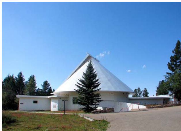
The Big Dome, later named the Evans Solar Facility.
