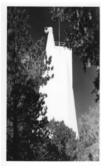
Fig 8. Upper left is a photo of Dick Dunn as he designs the VTT, not that his none beer hand indicates its height. Upper right and middle images are photo during construction, not sure OSHA would have approved the way those gentlemen are standing. Left: The finished DST extends 130 feet above ground and another 230 below. This allowed a very long focal length mirror. The light path from the entrance window seen on top to the primary and back to the ground level observing stations is evacuated to reduce internal telescope seeing.
