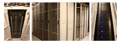
**Figure 6.3-1.** Photos of the new NISP Data Center in Boulder showing the data processing server rack (left), the POD in the SPSC Data Center that houses all four NISP racks (middle), and the expandable data storage cluster rack (right).
