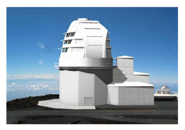
**Figure 2.** An artist's rendering of ATST at the primary site on Haleakala. Elevation view is from the north. Note the white concrete apron located on the eastern (left) side of the facility that is used to reduce radiated thermal loading from the ground.
