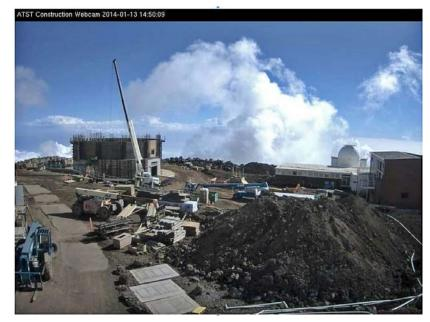
*Figure 5.2-1.* Site progress as seen in January 2014 (coudé pier is complete and the first level of the telescope pier is complete with forms set for the second level). The Utility Building is on the right hand side.
