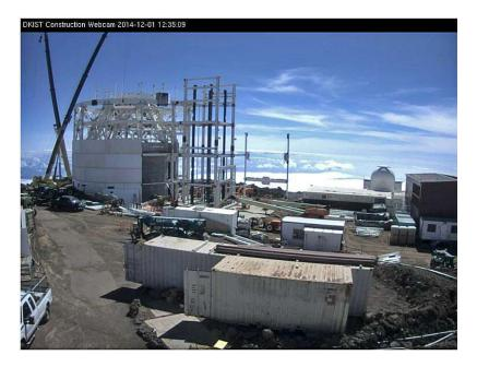
**Figure 5.2-2.** Site progress as seen in December 2014. Both piers are complete and the lower enclosure steel structure is in place along with a series of the pre-cast panels for the lower enclosure exterior. The platform lift steel is seen immediately to the right of the lower enclosure.
